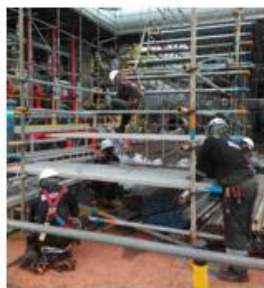
Erection of scaffolding as temporary platform
