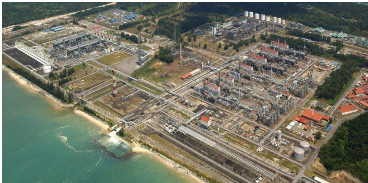
Figure 2. On-Shore Plant Facility
