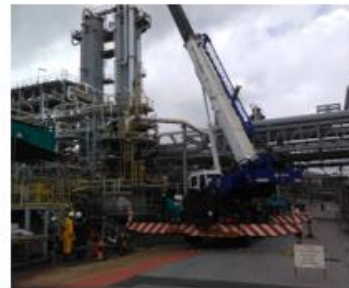
Critical lifting activity over live line with load more than 1tonne
