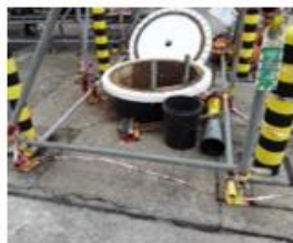
Confined space activity to do inspection work
