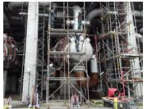
Erection of scaffold more than 5m height for paint job
