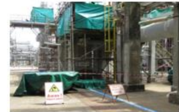
Hot work activity at height
