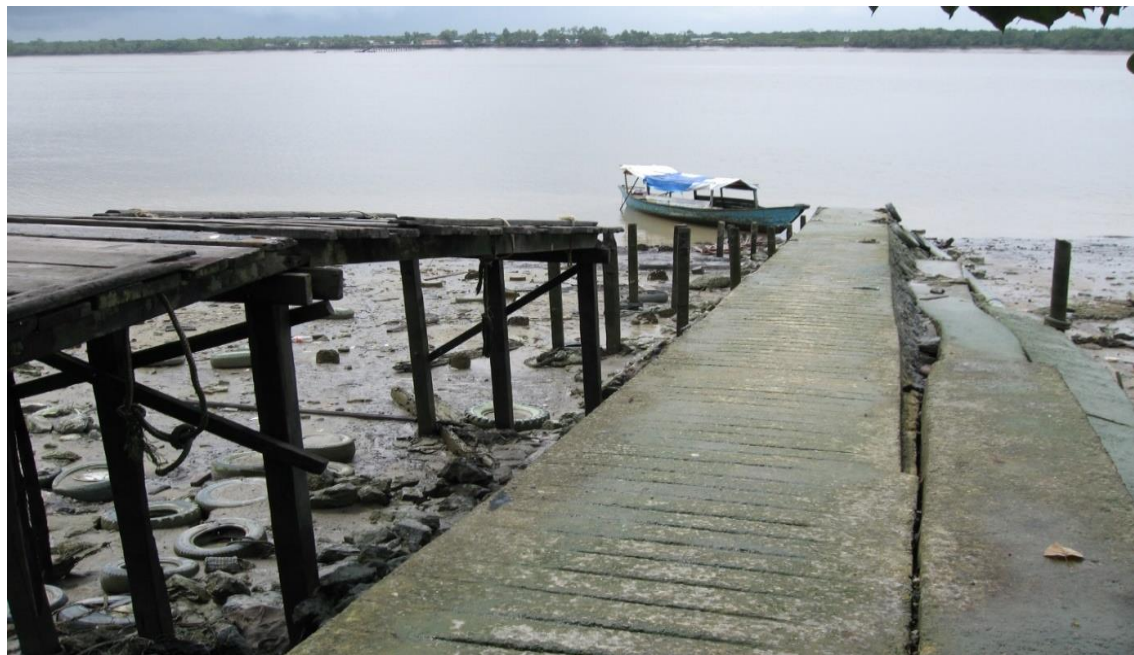
Figure 9 Old wooden jetty replaced by long cemented landing steps. Survey of landing facilities (SIWT, UNDP, 2008)
